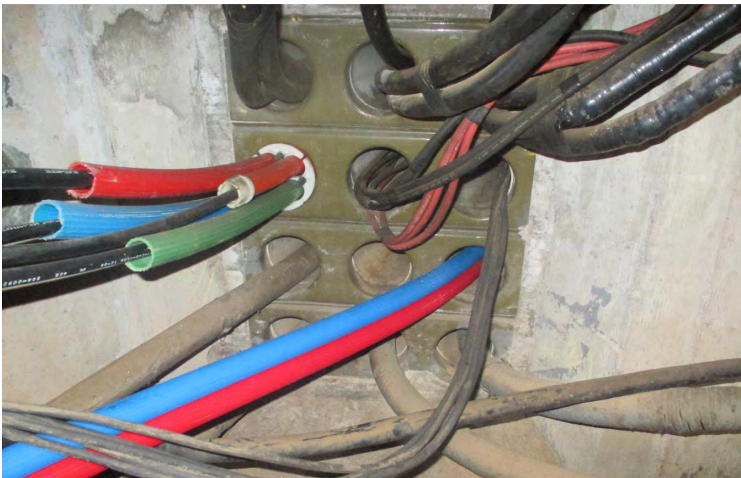
Figure 4.7 NU Network with Innerduct and Cable
